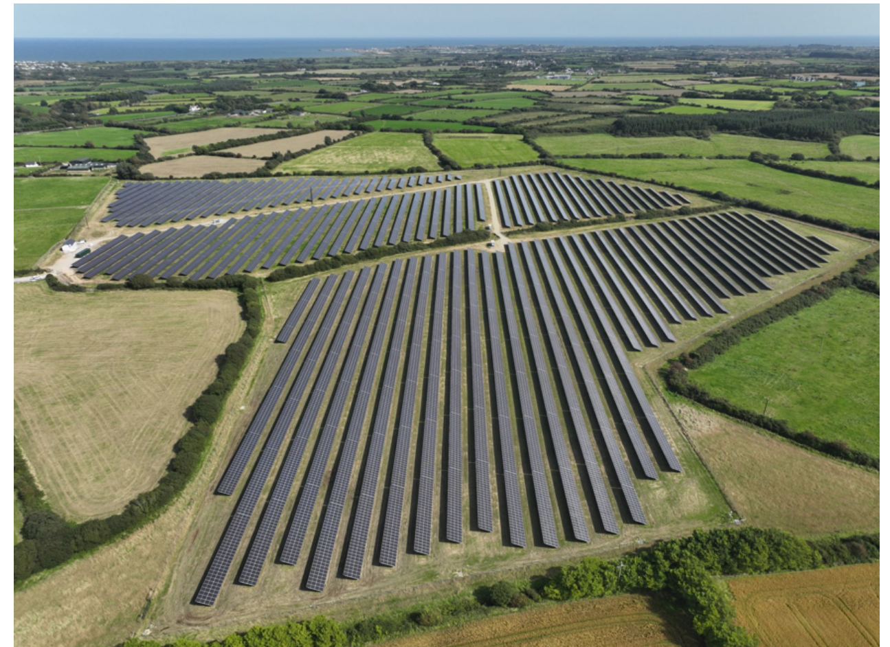
Blusheens Solar Farm, Co. Wexford
